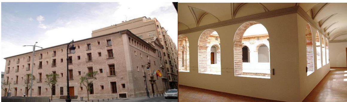
Figure 17. (Buildings of UCV in the city centre)
